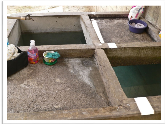
This concrete structure is called a "pila" and receives all the water coming in from the town. It's tepid, and is the only source of water in the whole house. I keep it full at all times, just in case we don't have any water for a day or two! It's here that I wash dishes and do laundry.
