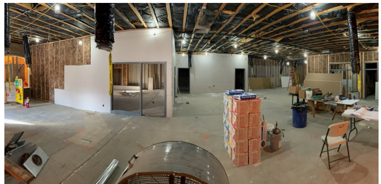
July: Beginning stages of drywall after completion of plumbing, electrical and framing.
