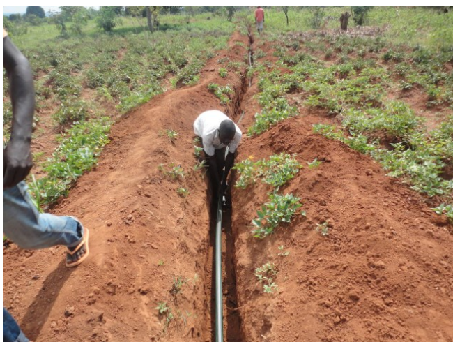
Water piping the entire 6 Km length
