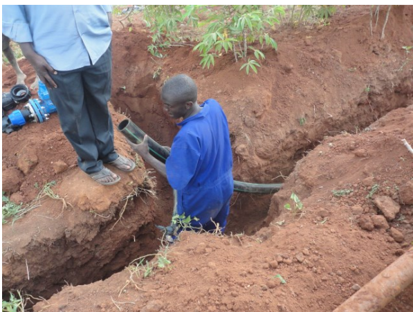
NWSC Engineers connecting the Buffujja line on to the mains NWSC Supply line.
