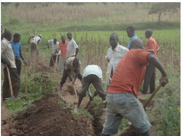
Clearing the Clogged up areas along the line
