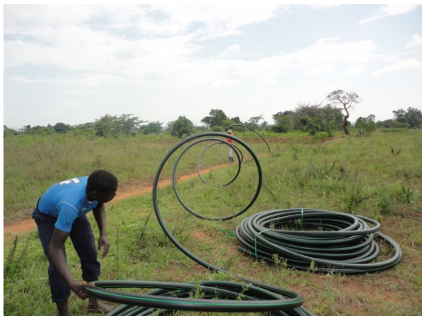
Un folding the water pipe ready for installation
