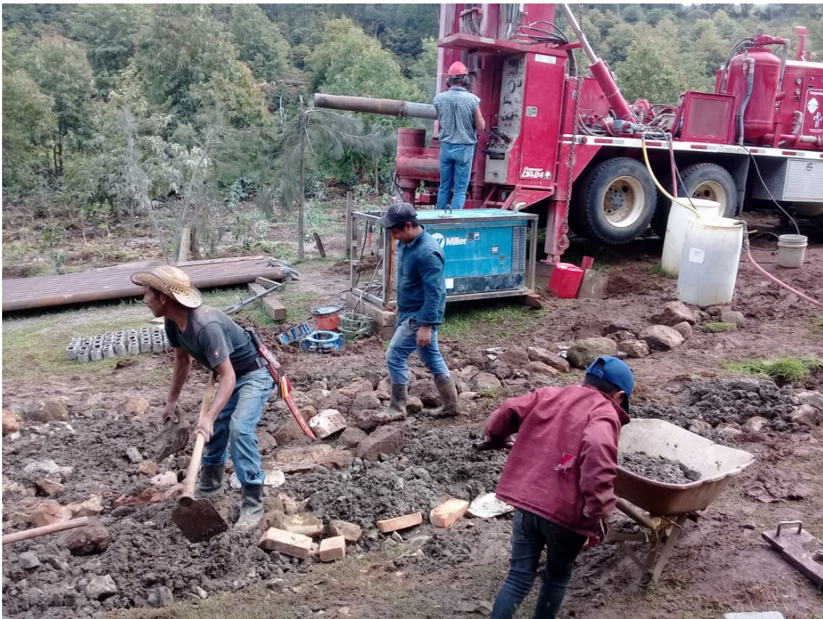
Building a new well in El Carrizal
