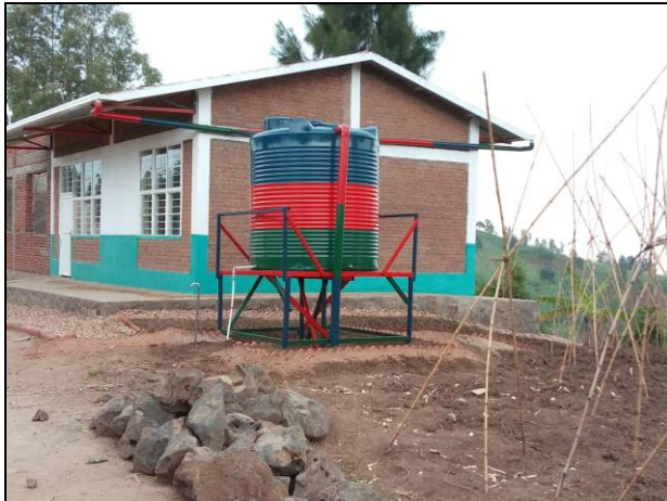
Kinigi Primary School Water Tank – installed adjacent to the Nursery School Classroom, harvesting rainwater from the classroom roof. Photos courtesy of Jill Fenton.
