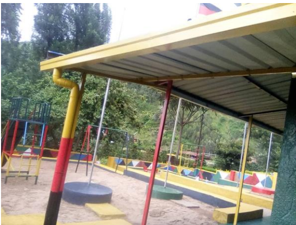
New and repaired rain gutters, paint inside and out and landscaping to assist water drainage.
