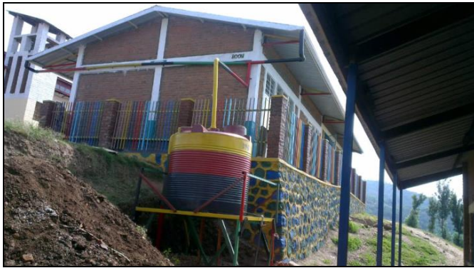
Busoro and Rambo Primary Schools – 5,000 litre water catchment and storage tanks at each of the new nursery school classrooms. Photos courtesy of Jill and Greg Fenton.
