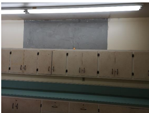
Repair work on wall from roof leak. Note the old fluorescent light fixtures
