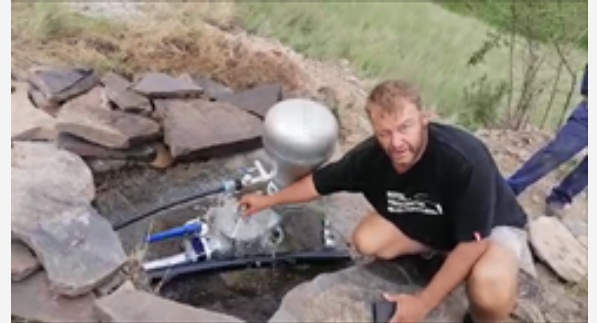
The pumps in action
