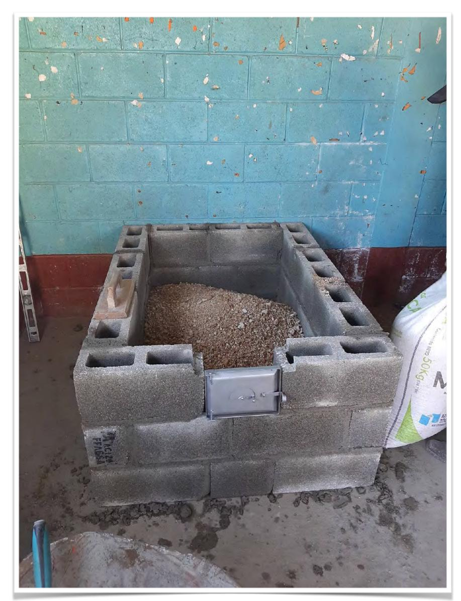
The mason builds a framework of cement blocks filled with sand and gravel.
