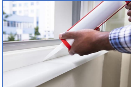
Caulking and weather stripping
