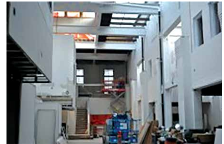
Eva's Phoenix construction site
