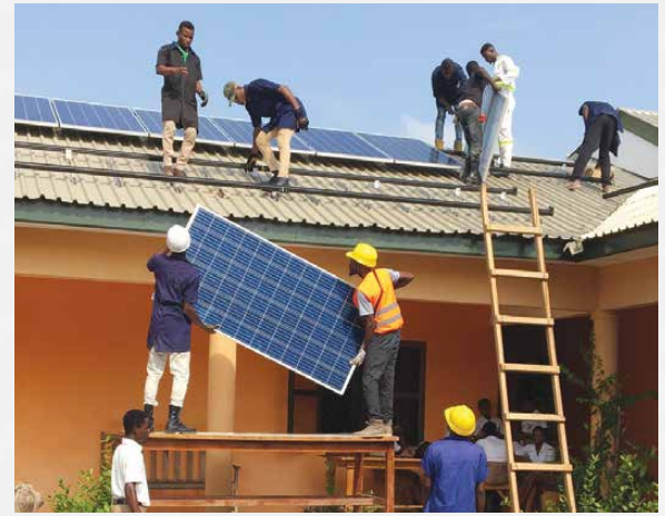
Getting it done – electrical students at work
