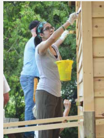
Staining the new cabin
