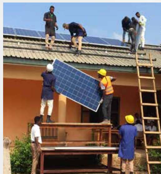
Raising the 127 panels to the roof
