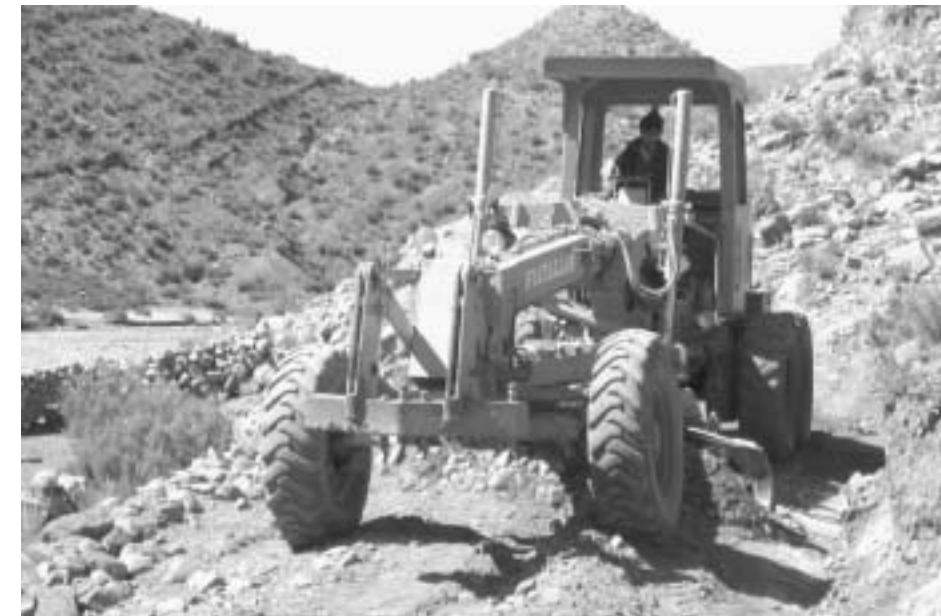
Connecting communities: Mano a Mano heavy equipment at work
