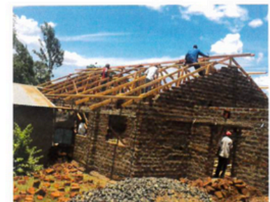
Constructing FOM church at Sitatunga
