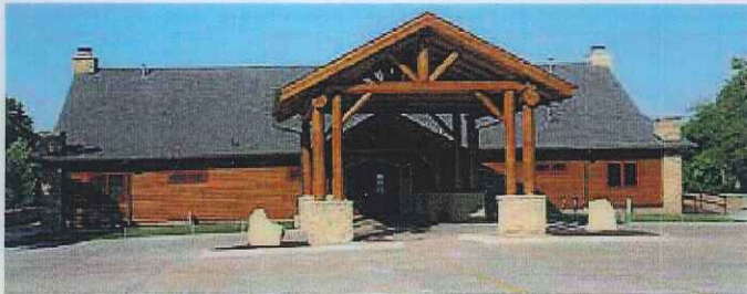
The refurbished Eagle Point Lodge.
