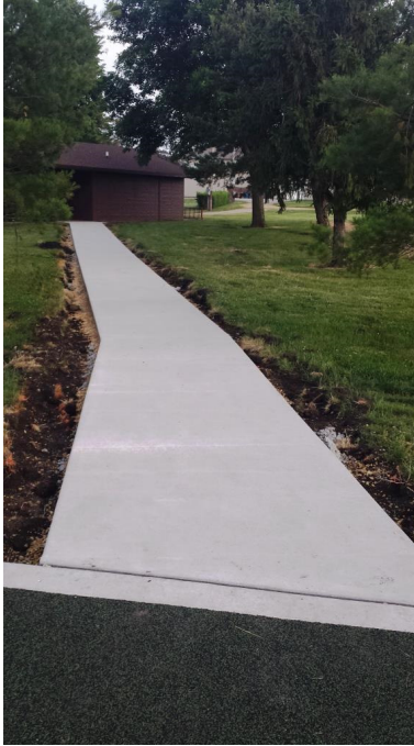
AND All the Concrete Work
