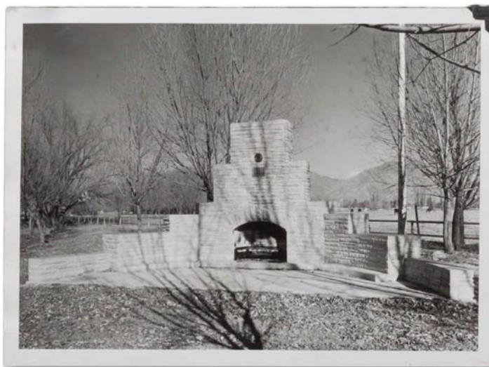
Willow Park public fireplace, constructed by Logan Rotary, stands complete, October 12, 1949. Logan Rotary Club papers, MSS 234, Box 8, Scrapbook 1.
