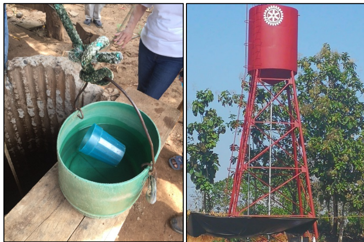
Typical residential water well in the community of La Vega and how water is removed from the well. Proposed water tank at La Vega.
