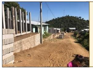
Connie's note: This is a view of the worksite when they arrived. The local men prepared the house foundations, which are terraced, and set the poles in place. Further down the hill you can see two more houses to be built with poles in.
