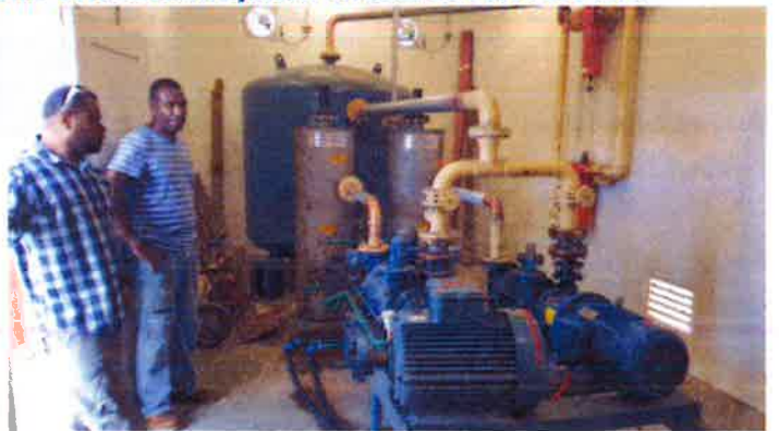
The BHS suction system installed at VCH Port Vila
