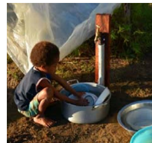
After: 1000 metres of poly pipe laid and 10 taps installed
