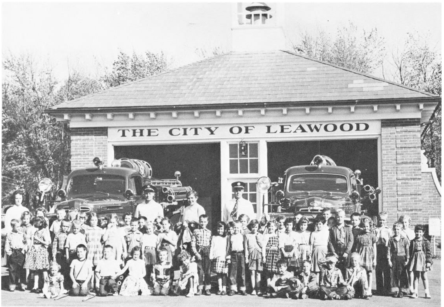
The Fire Station was constructed in 1951, and children were welcome to inspect the fire fighting equipment.
