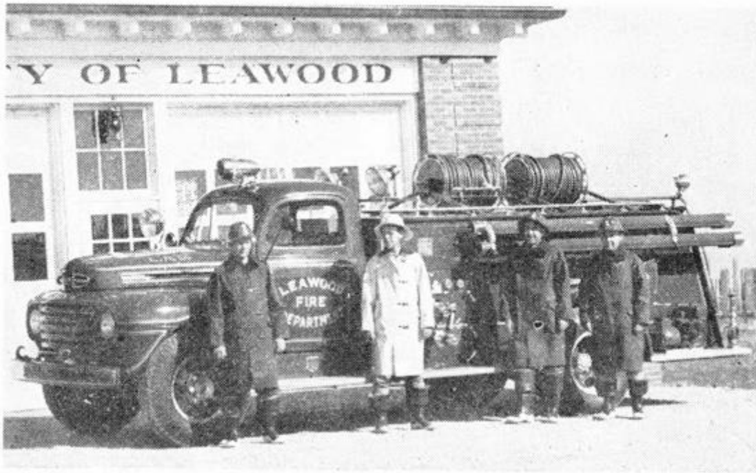
The first pumper was purchased in 1949. (Chief Brook Beatty is in Center.)
