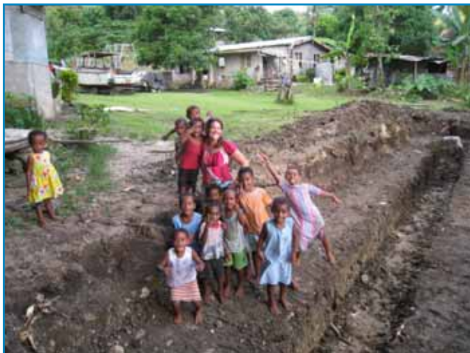
Top, current sanitation systems in Fijian villages. Above, Holly Gittlein with some of the children who will be able to live healthier lives because of the project. Next column, workers on the banana trenches that will filter and cleanse wastewater that flows to the sea. Next page, workers inspect banana trench. (Photos provided by Holly Gittlein)
