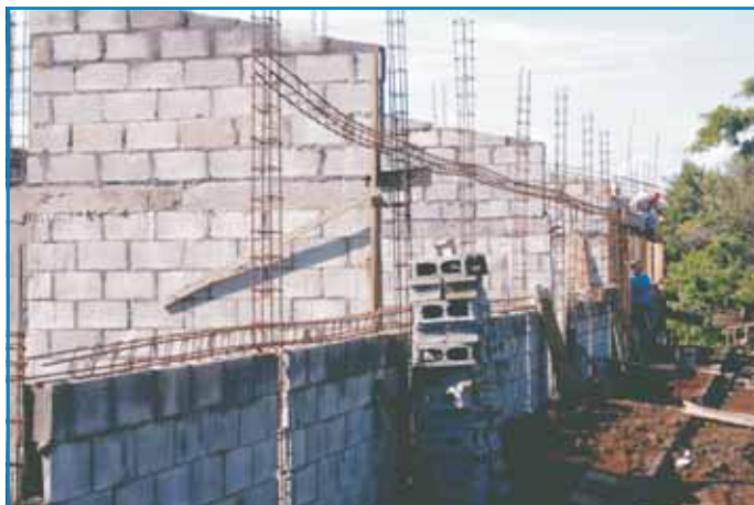
New school under construction
