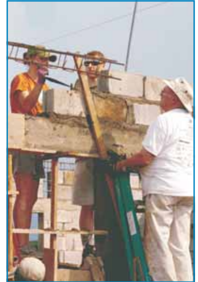
Al Fedoriak, PDG District 5010, laying block.
