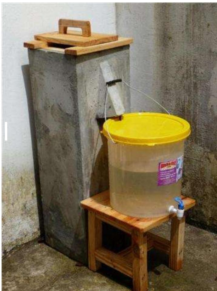
Here is a picture of the filter. This shows the 5 gallon safe water container, two of which are supplied for each home to receive the clean water, store it, and dispense the water safely from a tap. The tap assures that no contamination will occur from people dipping into a container with their hands or from airborne bacteria, pests or animals. Wilson, the designer of the table used to hold the container, was also a student in the training class in March and would like to start his own business.
