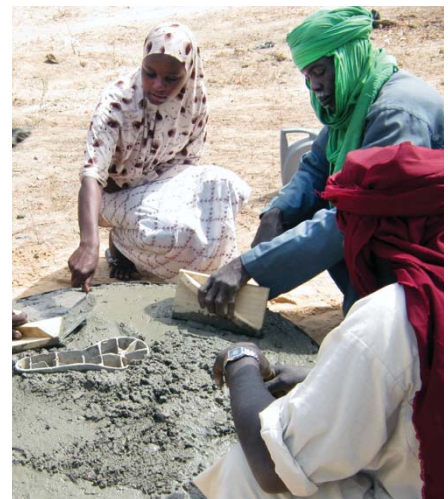
Artisans in a Niger World Vision project area learn to make concrete sanitation platforms for latrine construction.
