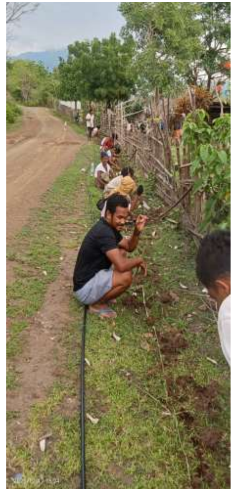
Top left: John Wotherspoon and Paul Jupp with southern coast villagers Above: Preparing to lay pipes
