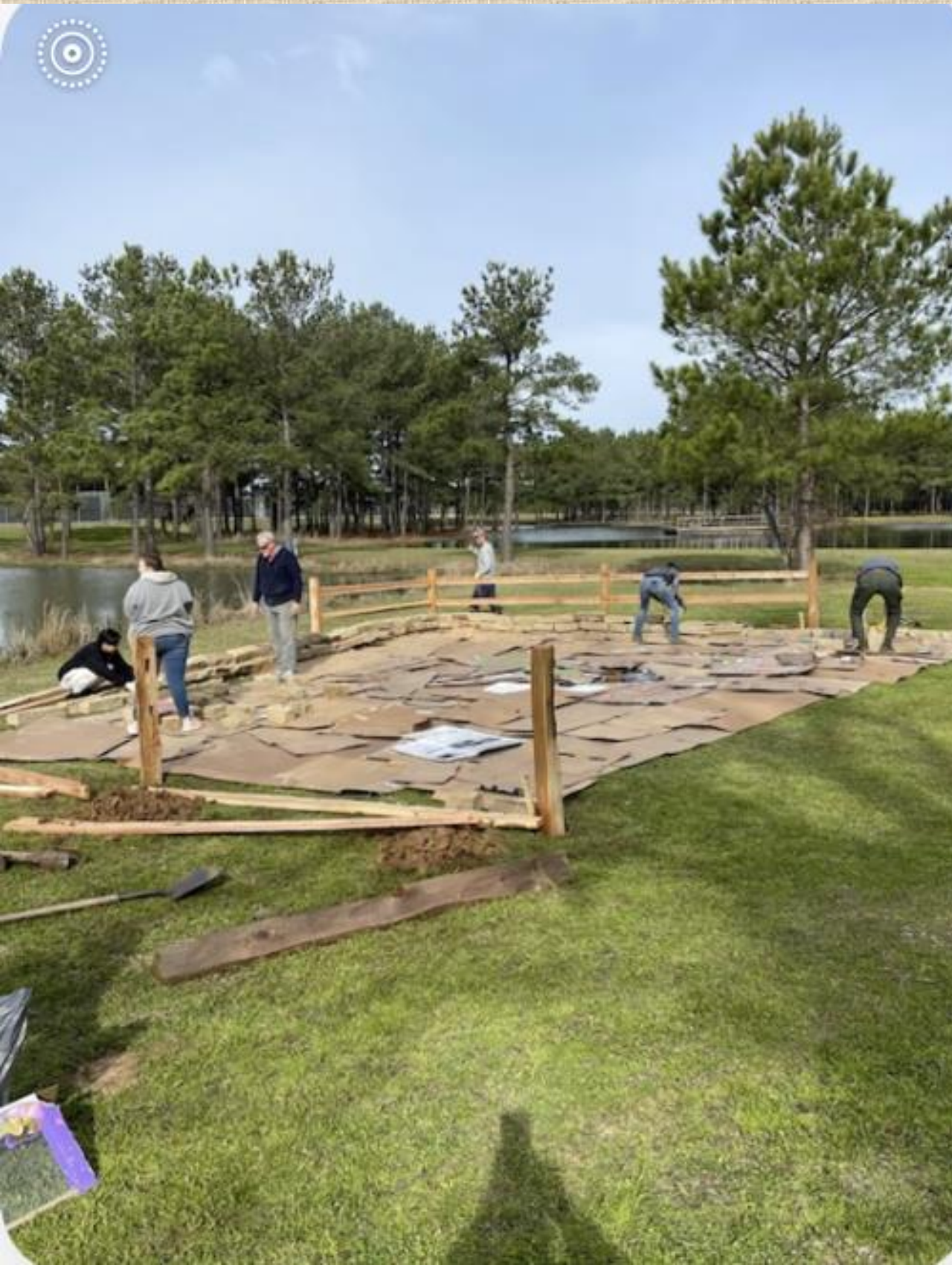
Laying Stone and Grass Barrier
