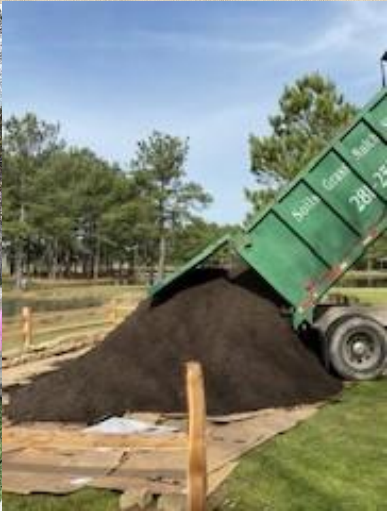
25 yards of Topsoil
