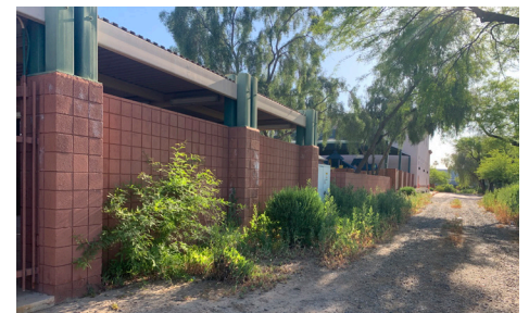
Photo shows some of the weeds behind the YMCA building.
