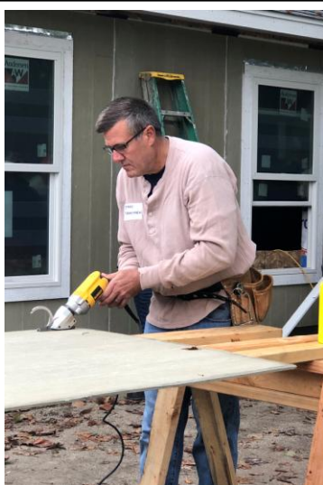
Stan Rasmussen cuts siding outside the Habitat home.
