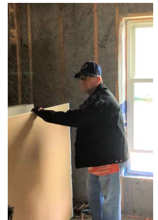
Wayne Whitney moves a section of sheetrock.
