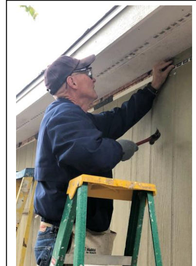
Mike Chapman nails siding trim to the Habitat for Humanity house.
