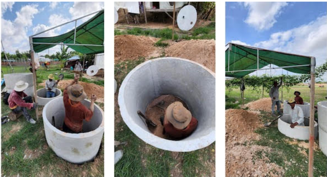
Digging in the concrete tanks for the septic system.
