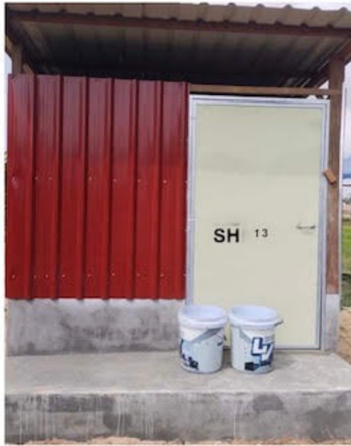
The height above ground is to allow for heavy rain in the wet season.
