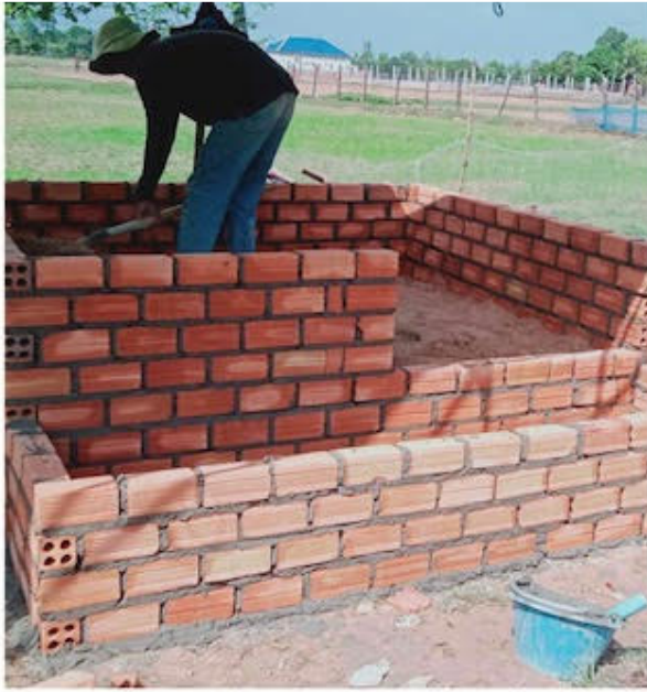
Building a brickwork base for the washroom toilet.
