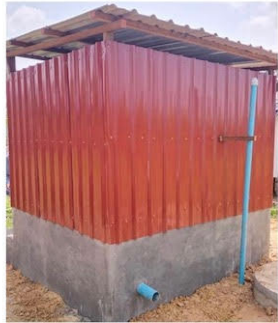
The height above ground is to allow for heavy rain in the wet season.
