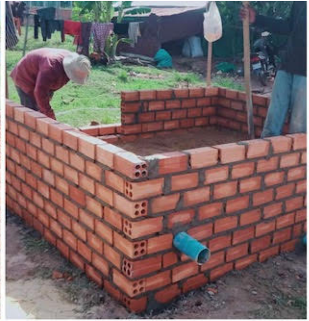
Building a brickwork base for the washroom toilet.
