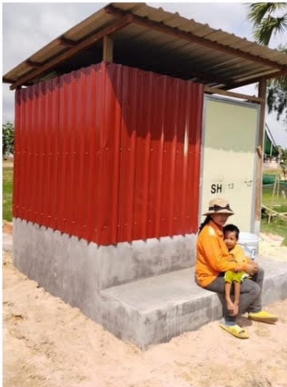
The height above ground is to allow for heavy rain in the wet season.
