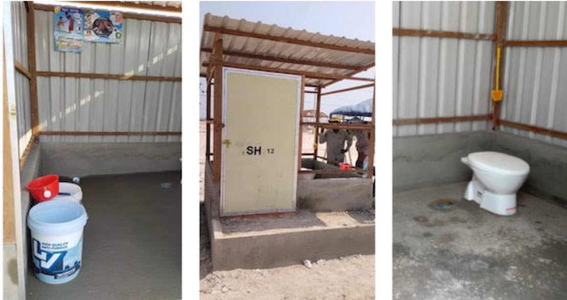
The walls and roof are made of 'colorbond' style steel sheets. The toilet door is a pre-made steel framed structure to ensure longevity.
