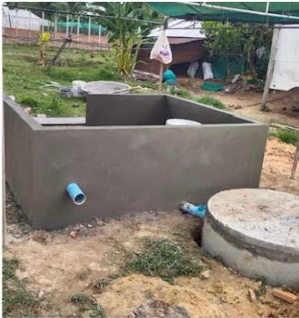
Rendering the brickwork ensures a waterproof washroom base.
