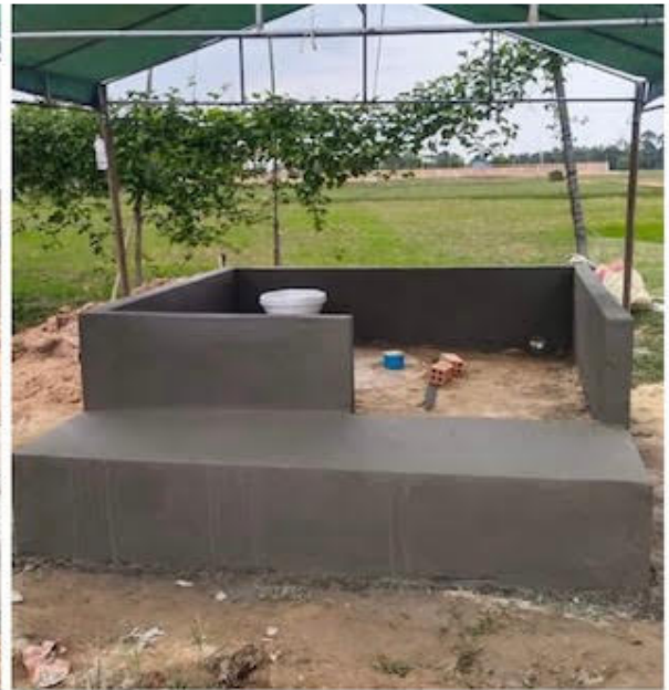
Rendering the brickwork ensures a waterproof washroom base.
