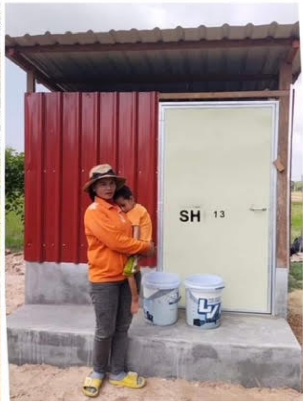
The height above ground is to allow for heavy rain in the wet season.
