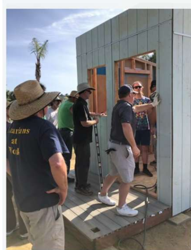
Cottage Build Spring 2024
