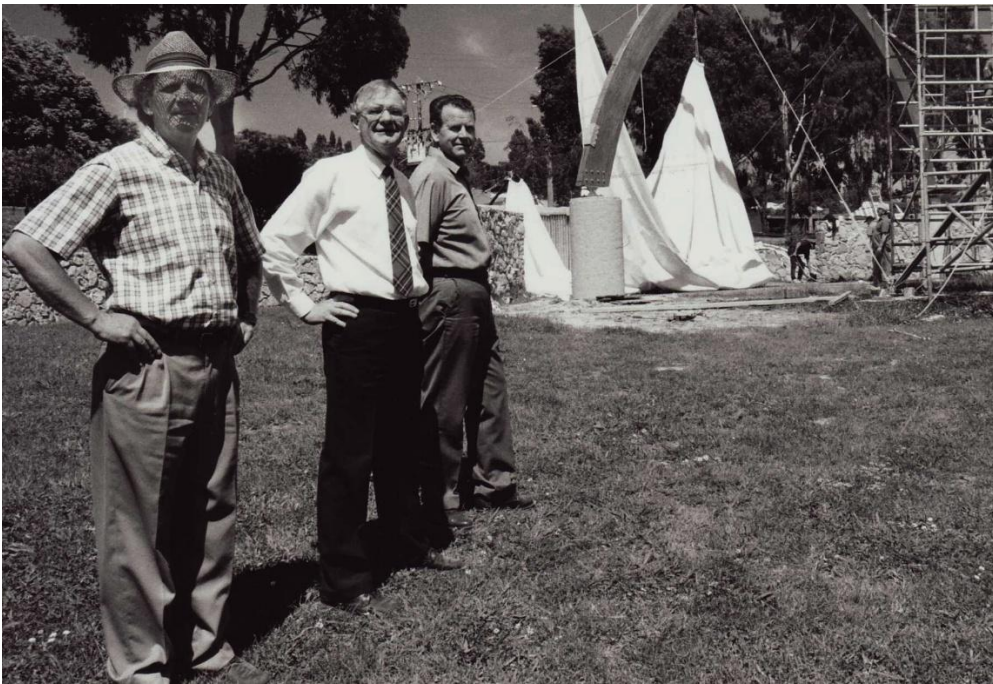
Architect Auden Pedersen with President Rob & Keith Pretty in front of the construction of the Drouin Sound Shell
