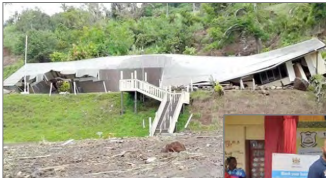
Dreketi School (damaged by Cyclone Winston).
