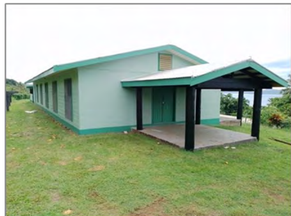
Views of the completed refurbishment work.
