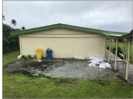
The existing concrete pad shown before work commenced.
