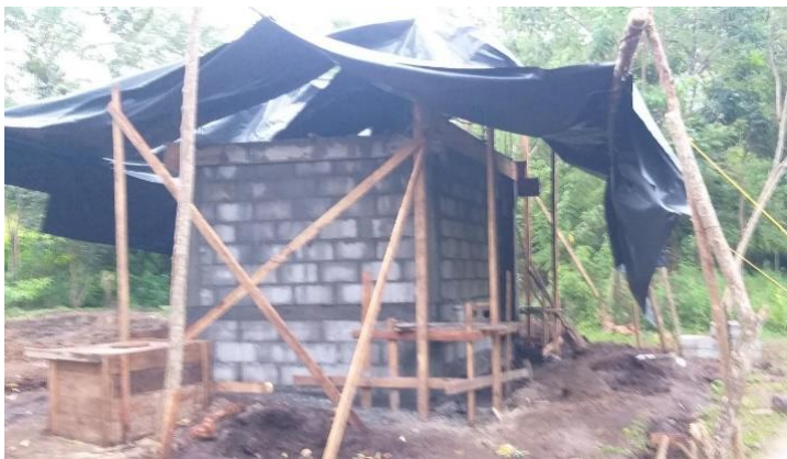
Construction of pump house – in the rain
