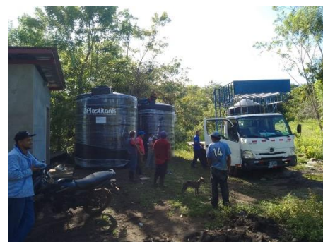
Delivery of the retaining tanks
