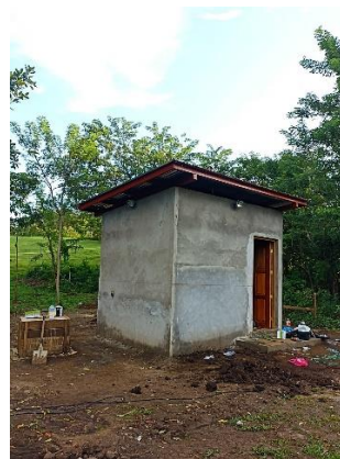
Completed pump house
