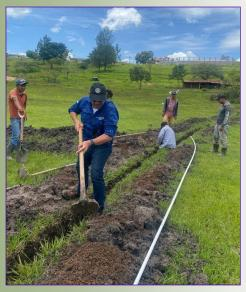
Construction began in April of 2022. Since our last update in June, materials for the distribution system were delivered and the community came together providing labor to dig a 13 kilometer (8.07 mile) trench and install 3/4 inch **PVC** piping from the pump to the
