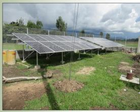
at their own expense to work with the community on the project and inspect the water tank installation. The solar panels shown above are one of the first arrays installed on our projects and are intended to provide some of the power for the water pump reducing energy costs.
