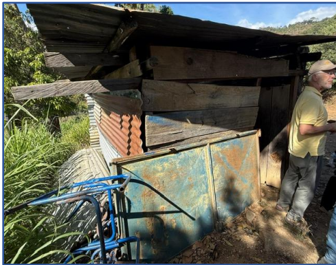
The existing kitchen has partial walls, an adobe stove and dirt floor
