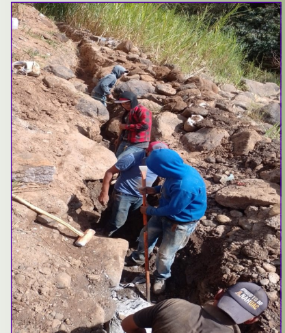
Community members volunteer their labor trenching for a distribution line
