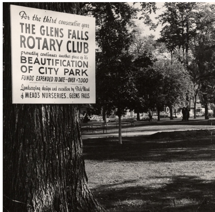
City Park Rotary sign
