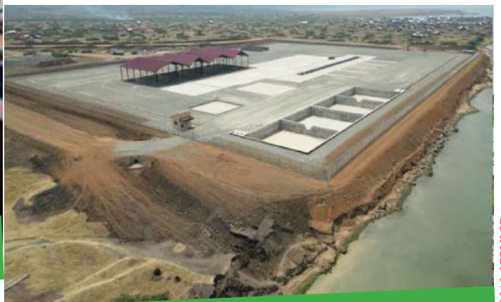
EXCEL CONSTRUCTION LTD. - UGANDA
