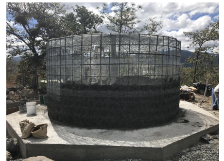
The new water tank half up.
