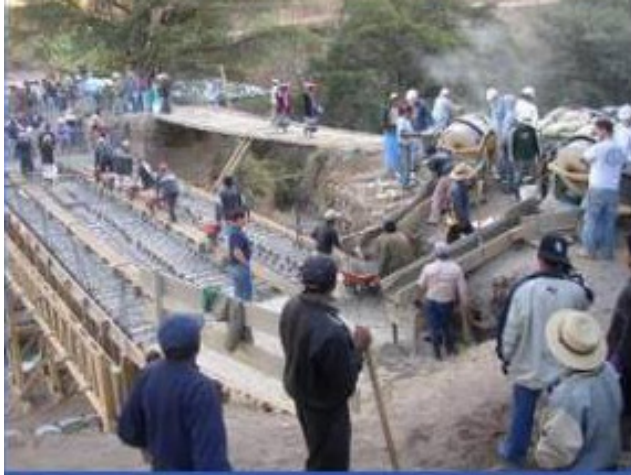
Building a bridge in Guatemala
