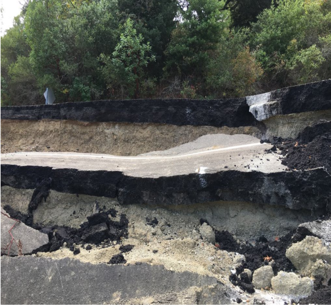
DOWN SLOPE VIEW OF SLIP OUT
