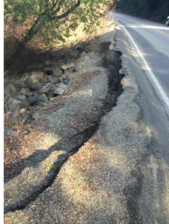
Norris Canyon Shoulder Slip-Out Before and After
