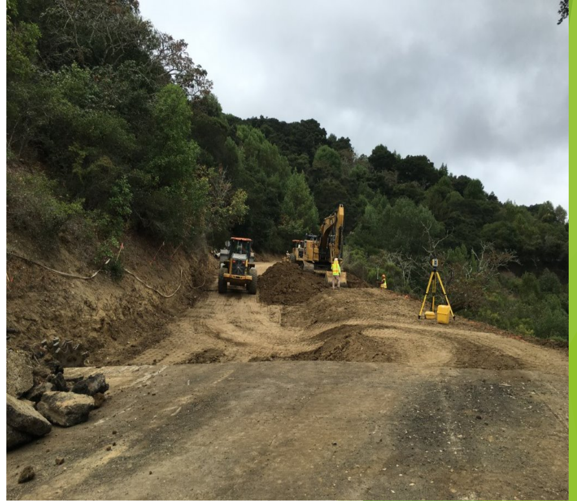
WORK BEGINS WITH ROUGH GRADING
