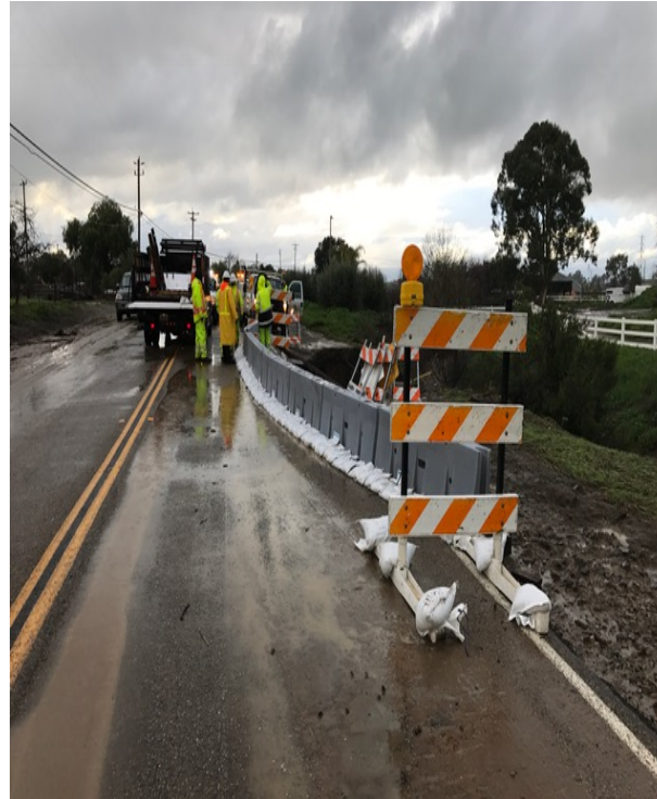
Barricades installed for traffic control while Tesla Road way was repaired. (after)
