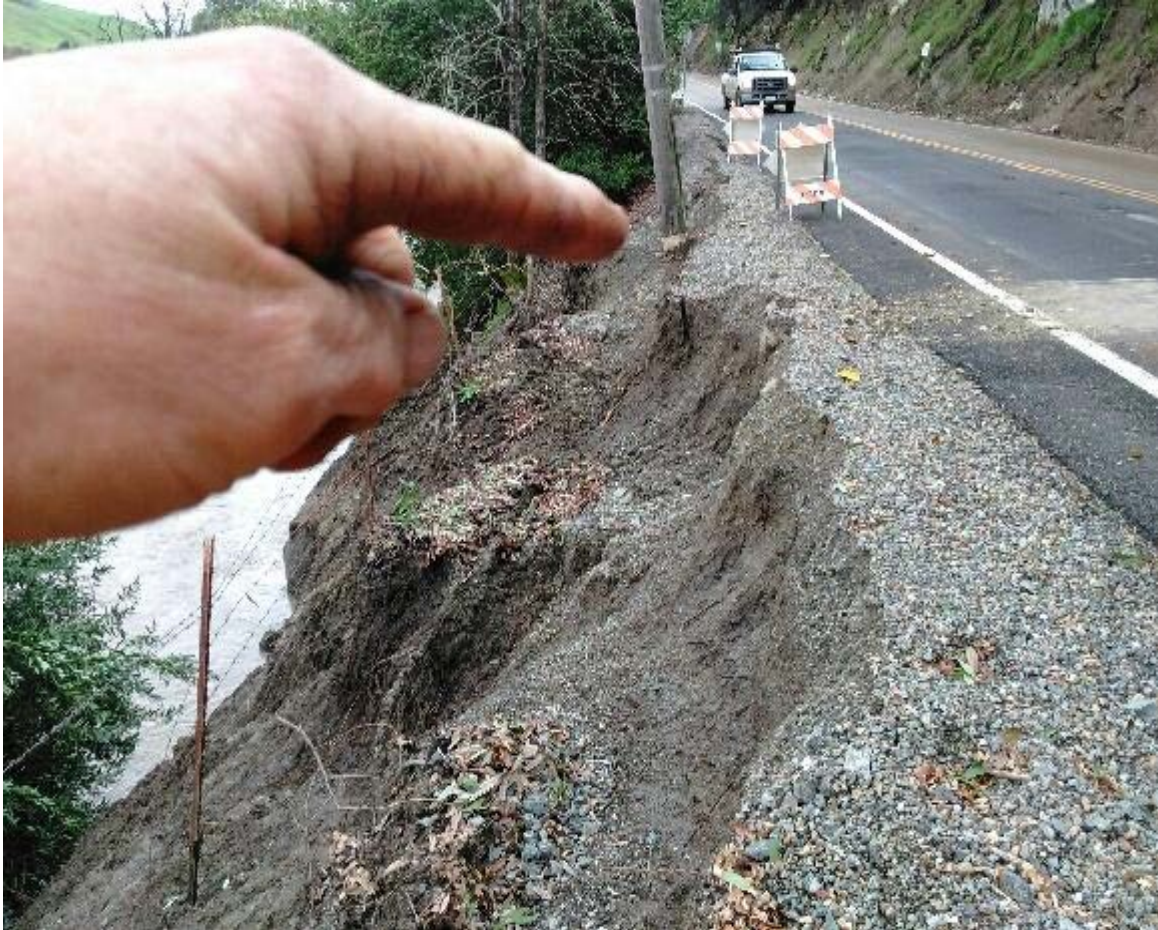
Foothill Road, Pleasanton Slope Failure at mile marker 6.92 (before)
