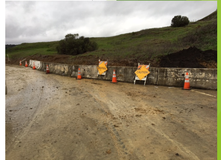
Slope protection (barricades) were installed and Koopman Road is open with one-lane traffic control (after)
