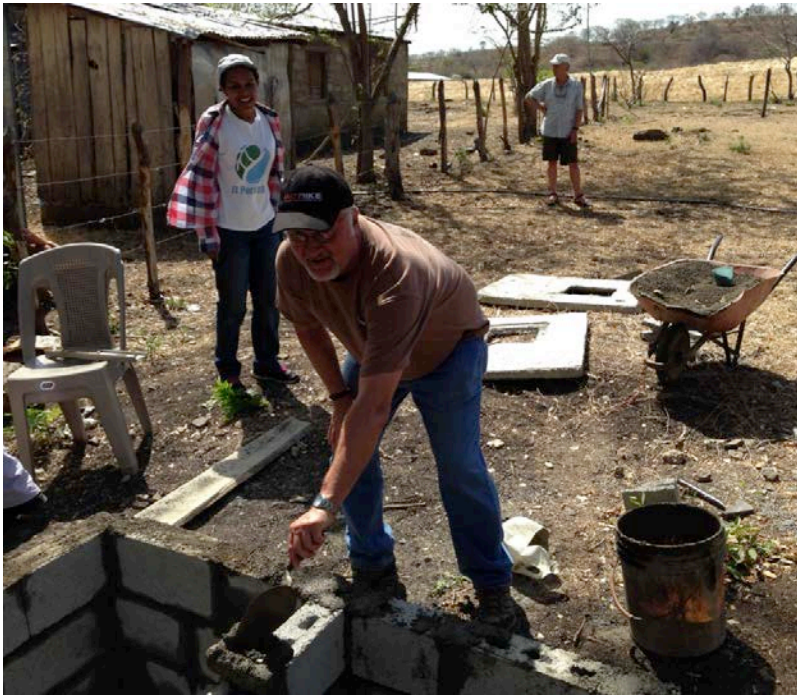
Figure 10. Bob Kemp Mortaring Bricks for Latrine at El Tule
