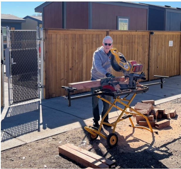
Tom Cella hard at work building SOS housing. 04/24
