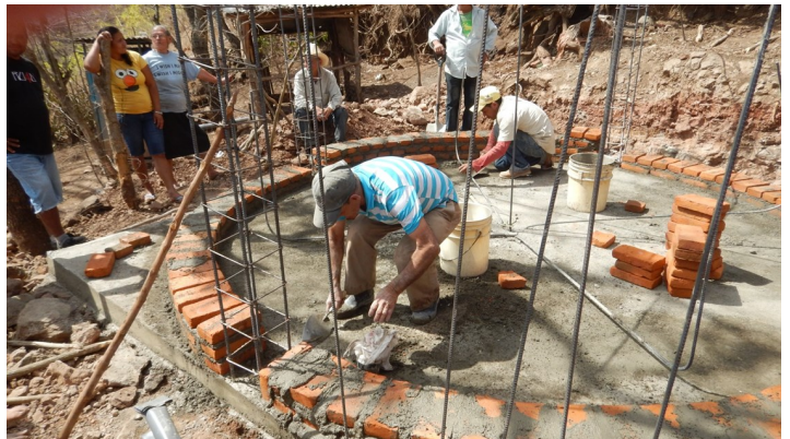
APTU WATER TANK BEING CONSTRUCTED AT THE HIGH POINT IN THE VILLAGE
