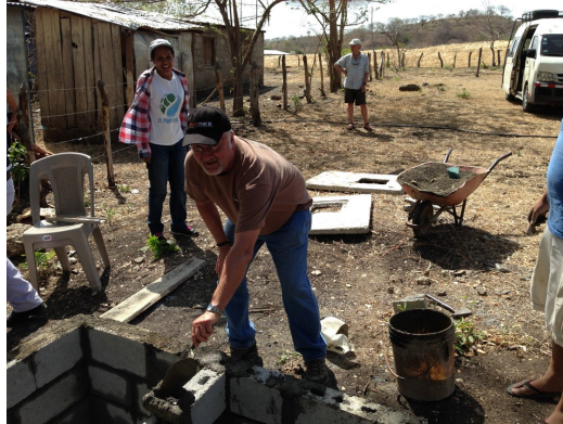
BOB KEMP MORTORING BRICKS FOR DOUBLE PIT LATRINE AT EL TULE
