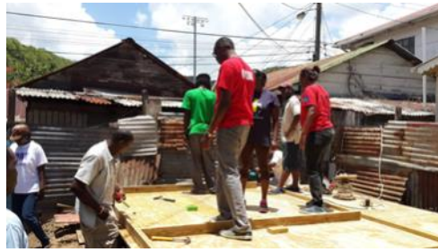
In no time the side panels were cut and assembled
