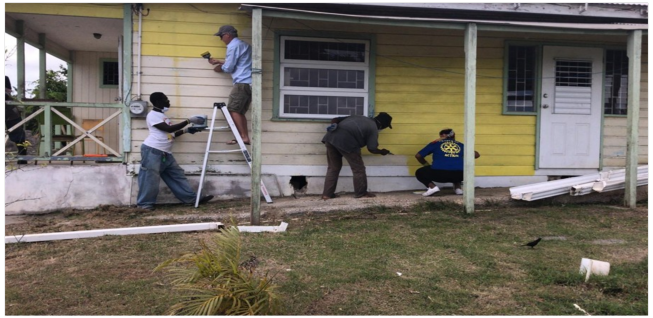
BoView House being painted
